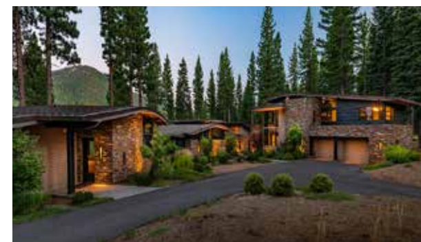
Home 368 - $9,295,000 6,365 Sq Ft / 5 Bedroom - 5.5 Baths Ward-Young Architects / Jones Corda Construction
